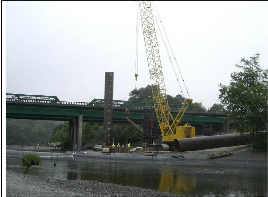
**Figure I.3-57 Pier 3 Location and Water Bladder**
