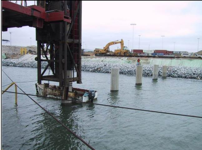
**Figure I.5-6 Driving of 24-Inch Octagonal Indicator Piles at Port of Oakland Berth 22. Pile being driven is in Row A, while Row E is at the shoreline.**
