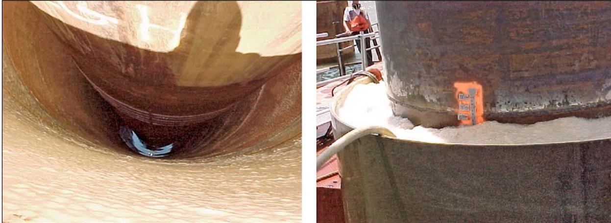
**Figure 2-29. Confined Air Bubble Curtain System Used at an Isolation Pile at the Benicia-Martinez Bridge**
