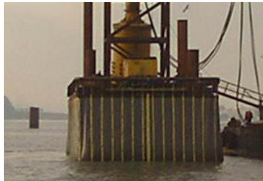
**Figure I.9-4b Proprietary Fabric Air Bubble Curtain (Proprietary) Used during Driving of PIDP Pile 3**
