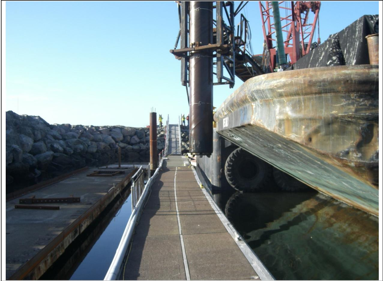
**Figure I.3-65 Placement of 24-inch Steel Shell Pile at the Crescent City Inner Harbor Dock**
