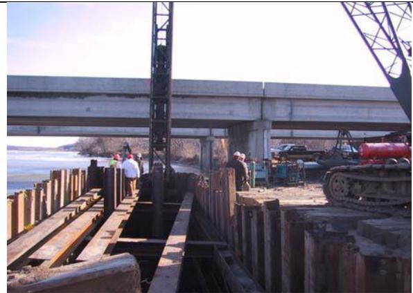
**Figure I.4-5b Dewatered Cofferdam Excavated below Water Level**
