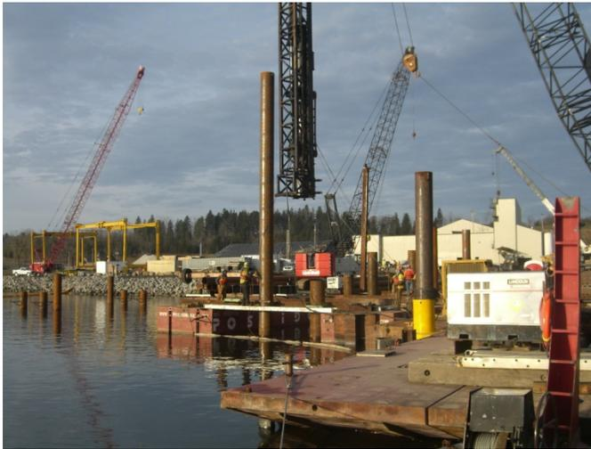
**Figure I.3-69 Pile Installation at the Straddle Crane Trestle**
