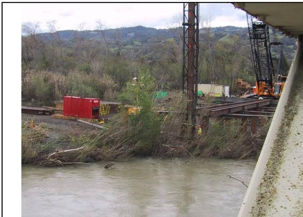
**Figure I.3-18a Trestle Pile Driven on East Bank. Note trestle piles extend back several hundred feet.**
