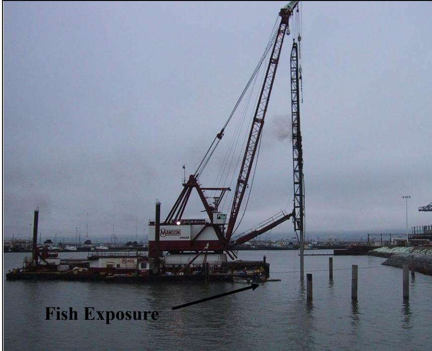
**Figure I.5-9 Pile Driving during Fish Exposure Study at Berth 22, Port of Oakland. Picture was taken 100 meters (330 feet) west of pile driving activity, while fish were being exposed at 10 meters (33 feet) from the pile.**
