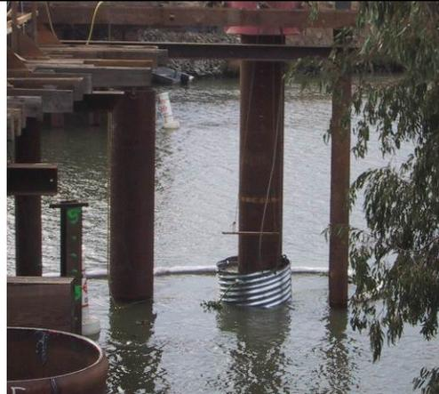
**Figure I.3-8 Casing for the Confined Air Bubble Curtain System**
