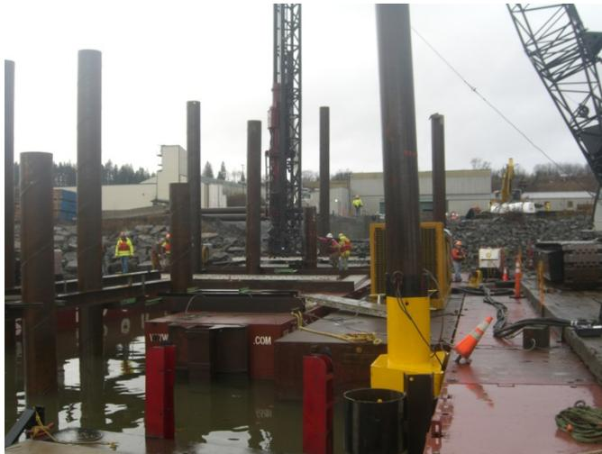
Figure I.3-70 Pile Installation at the Assembly Sled Trestle
