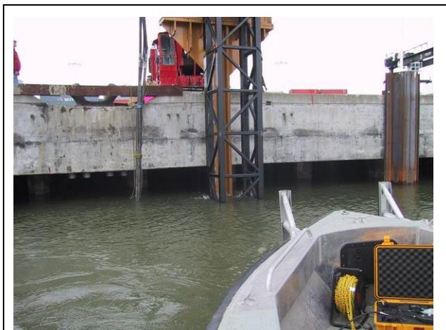
**Figure I.6-1 Driving of Steel Sheet Pile Underwater Using Hammer Follower**
