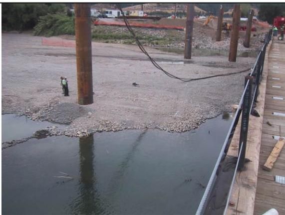
**Figure I.3-22a Vibratory Installation of a Bent 4 Pile with Bent 3 and Bent 2 in the Background**
