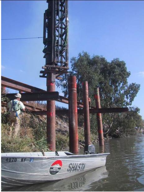
**Figure I.3-7a Driving 20-Inch-Diameter Piles near Shore**
