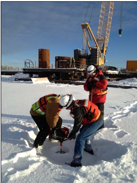
**Figure I.3-61 Crew Drilling Through Ice to Place Hydrophone**
