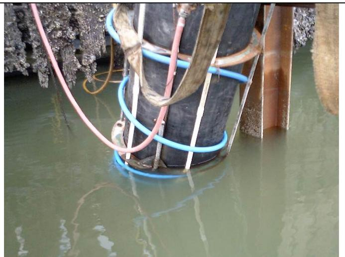
**Figure I.4-2b Close-View of Confined Air Bubble Attenuation System next to Vertical H-Pile**
