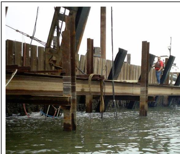
**Figure I.4-2a Impact Driving of Battered H-Type Pile with Attenuation System, with Vertical Thin-Walled H-Piles in Foreground**
