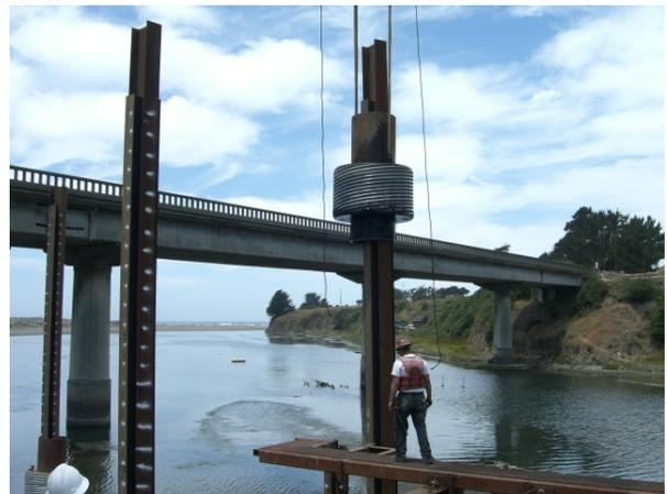
**Figure I.13-3d Isolation Casing Being Installed**
