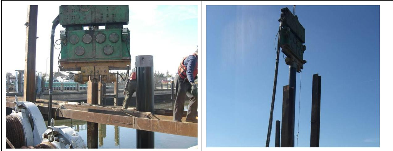
**Figure I.3-39 Pile Installation Using the ICE 66 Vibratory Driver**
