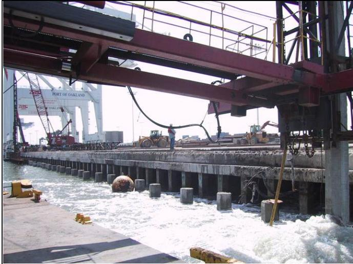
**Figure I.5-12 Driving of 24-Inch Octagonal Piles at Berth 32, Port of Oakland with an Air Bubble Curtain System to Attenuate Sounds**
