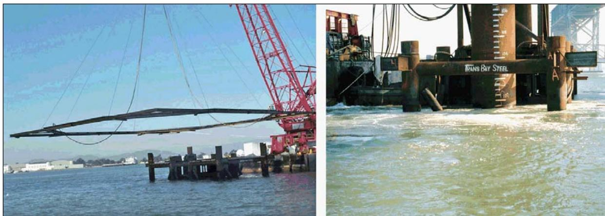
**Figure 2-20. Unconfined Air Bubble Curtain Systems**
