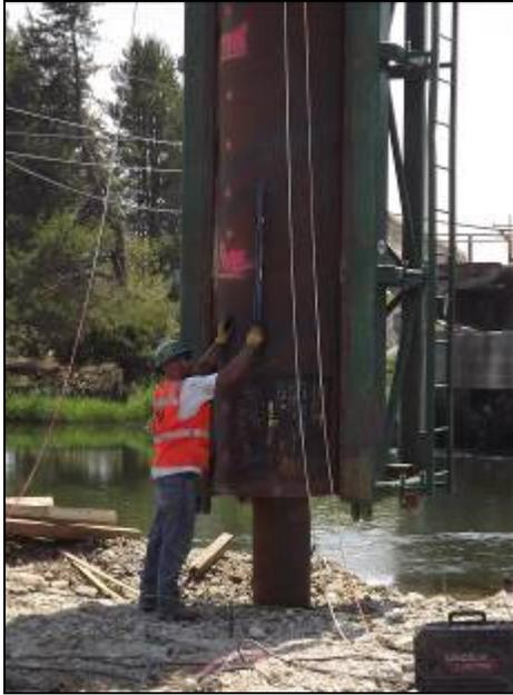
**Figure I.3-67 Placement of 36-inch Diameter Steel Shell Pile at North Payette River**
