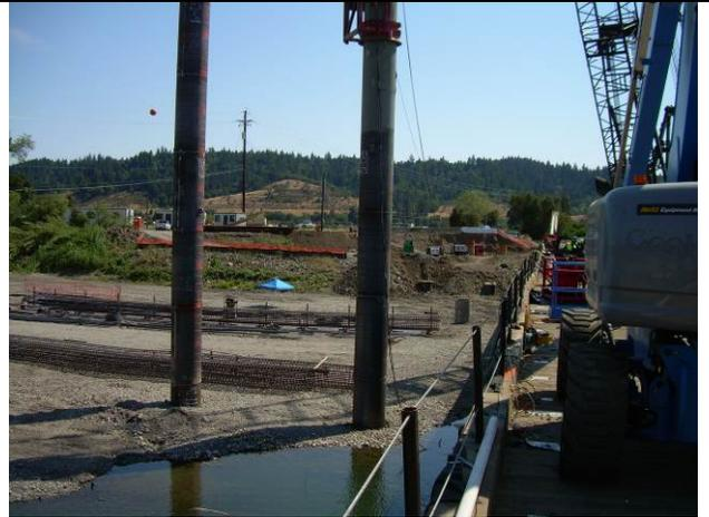
**Figure I.3-17b CISS Piles Driven to Support New Geyserville Bridge across the Russian River**
