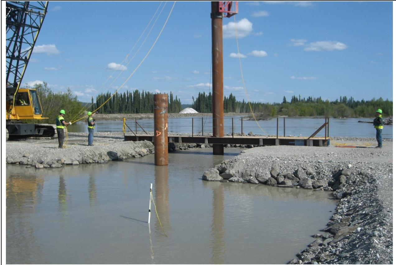
**Figure I.3-60 Driving of 24-inch Steel Shell Pile near Salcha, Alaska**
