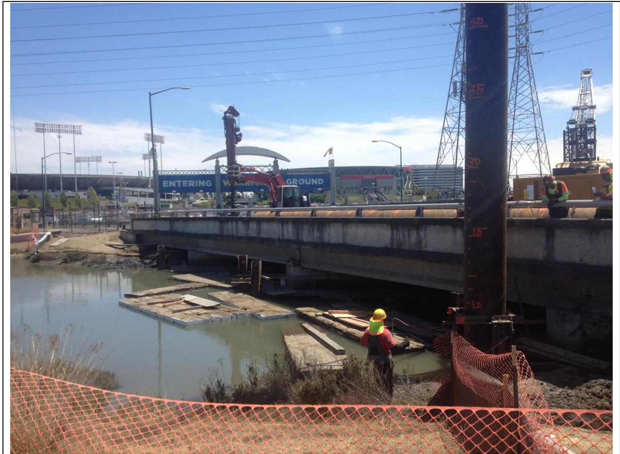
**Figure I.3-68 Placement of 36-inch Diameter Steel Shell Pile at Coliseum Way Bridge**
