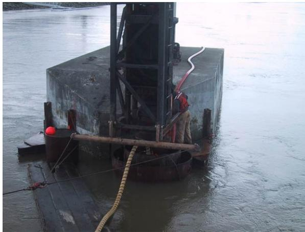
**Figure I.11-2c Double-Walled Attenuator – Humboldt Bay Bridges, Eureka, CA**
