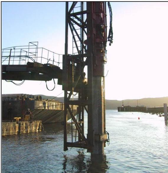
**Figure I.5-4a 24-Inch Octagonal Piles Driven at Amports in Benicia, CA**
