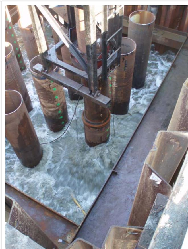
**Figure I.13-4 “Chaser” Attached to Diesel Impact Hammer Driving the Steel Shell Piles with the Bubble Ring on**
