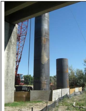
**Figure I.3-41 Impact Driving of On-Land Steel Pipe piles**
