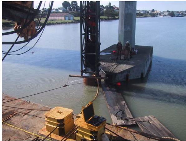
**Figure I.11-2a Driving 36-Inch-Diameter Pile in a 5-Foot Casing with Inside Bubble Ring – Humboldt Bay Bridges, Eureka, CA**
