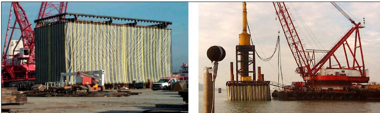
**Figure 2-28. Proprietary Confined Air Bubble Curtain System**
