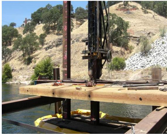
**Figure I.4-7a Impact Driving of In-Water H-Piles**
