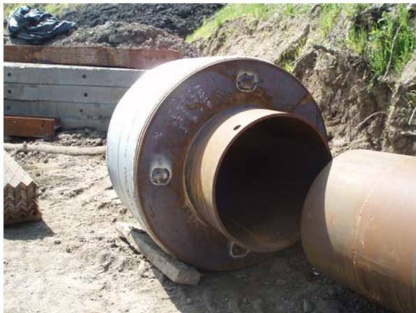
**Figure I.13-3c End View of Isolation Casing**
