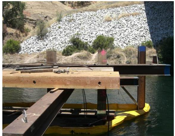
**Figure I.4-7b Impact Driving of In-Water H-Piles**
