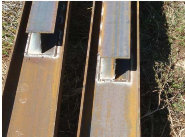
**Figure I.13-2 Modified H-Piles**
