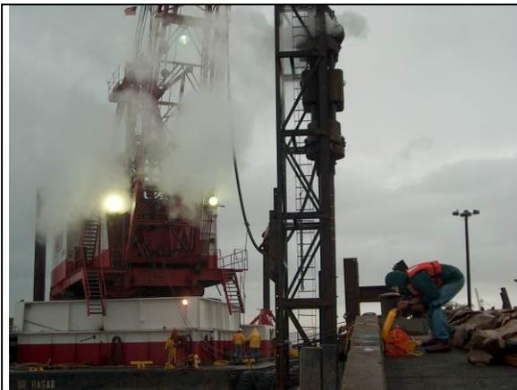
**Figure I.5-1a Driving of 16-Inch-Square Piles**
