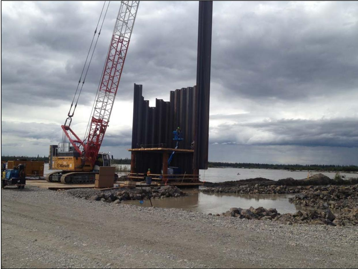
**Figure I.6-5 Installation of Sheet Piles**
