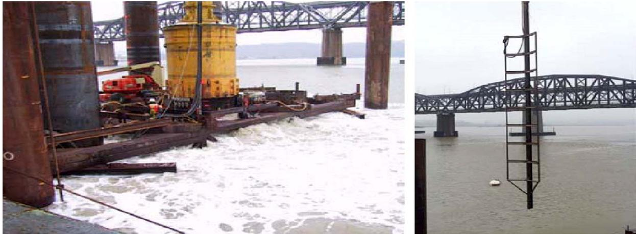
**Figure 2-25. Multiple-Stage Unconfined Air Bubble Curtain System**
