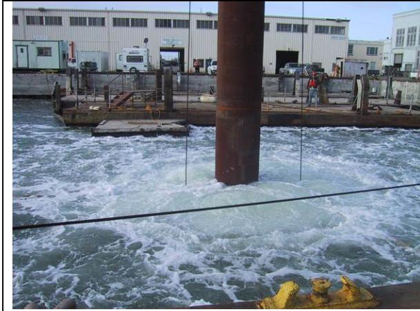
**Figure I.3-26a Driving 40-Inch-Diameter Piles with Air Bubble Curtain in Alameda, CA**
