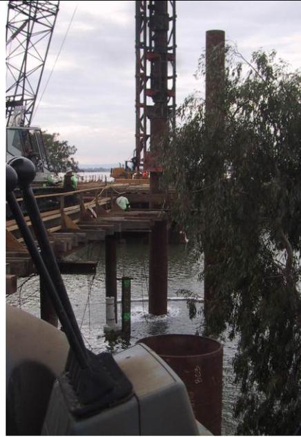
**Figure I.3-7b Driving 36-Inch-Diameter Pile with Attenuation**
