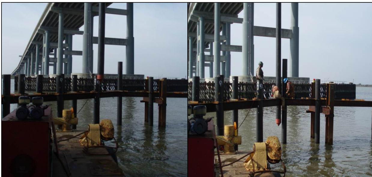
**Figure I.12-1 Typical Installation of 13-Inch-Diameter Plastic Piles**
