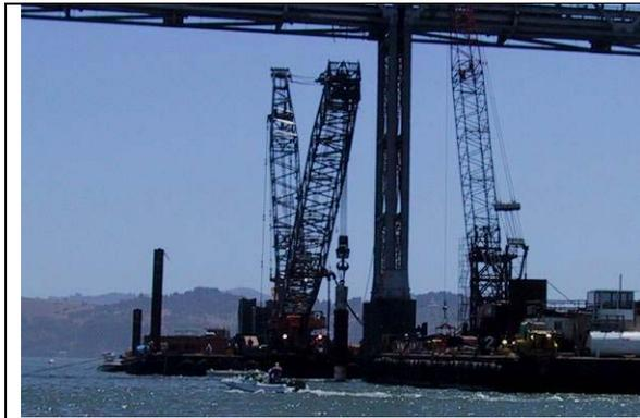
**Figure I.10-10 126-Inch-Diameter CISS Pile Being Driven Underwater at the Richmond-San Rafael Bridge**
