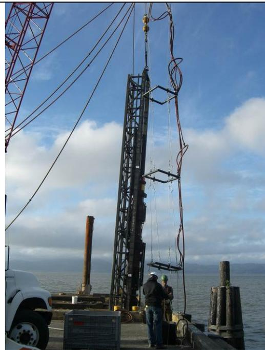
**Figure I.3-32 Deployment of the Bubble Rings—Tongue Point Facility Pier**
