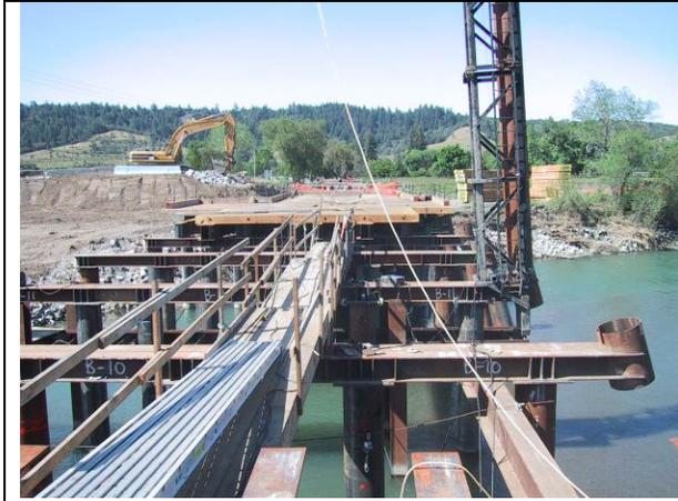
**Figure I.3-17a Construction of the Temporary Trestle across the Russian River**
