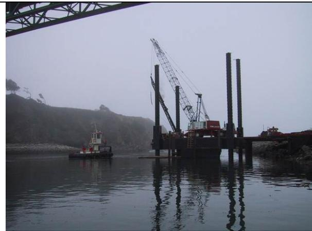
**Figure I.4-1b Impact Driving of In-Water H-Piles**
