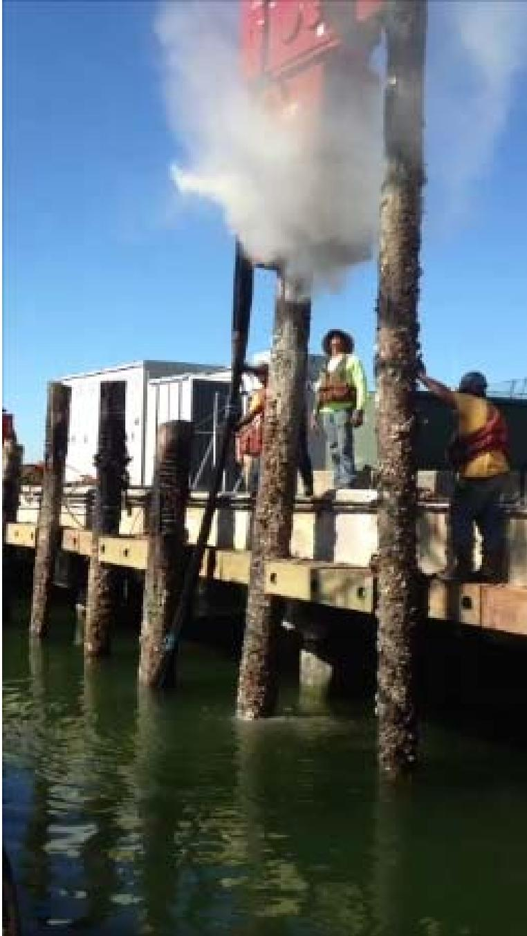
**Figure I.7-4 Installation of Timber Piles**
