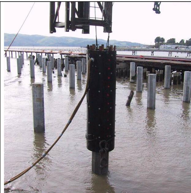
**Figure I.5-4b “Bubbleator” Used to Attenuate Underwater Sound**
