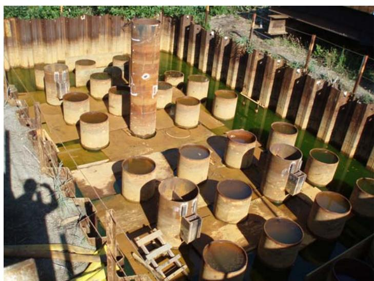
**Figure I.13-5 Pier 5 Steel Shell Pile Layout in Cofferdam Typical of all Pier Locations**
