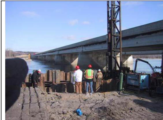
**Figure I.4-5a H-Pile Driving at the Platte River in Nebraska**
