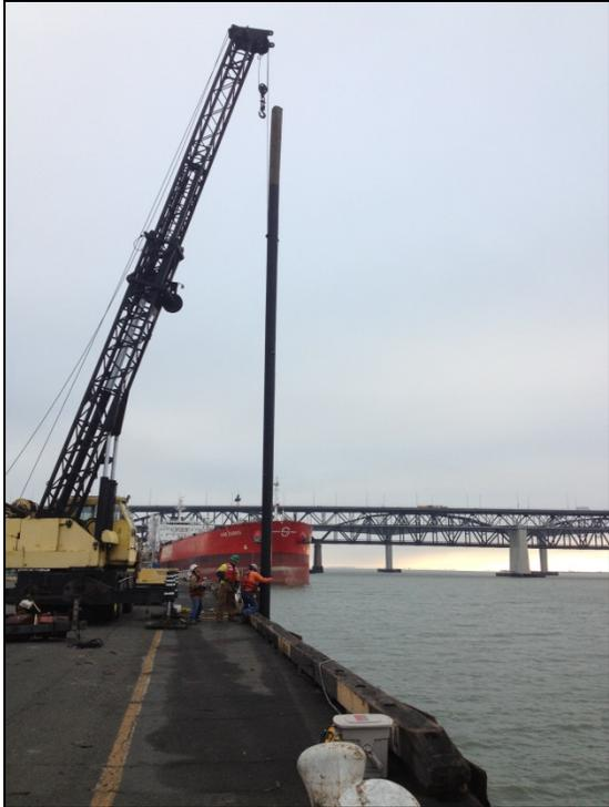
**Figure I.7-3 Wood Pile Installation at Port of Benicia**
