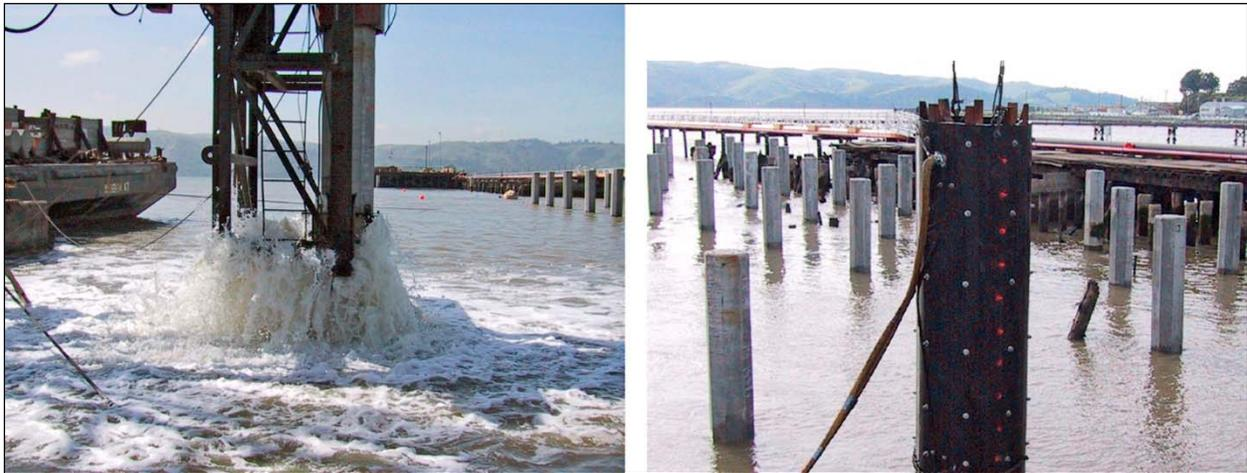
**Figure 2-31. Simple Confined Air Bubble Curtain System**
