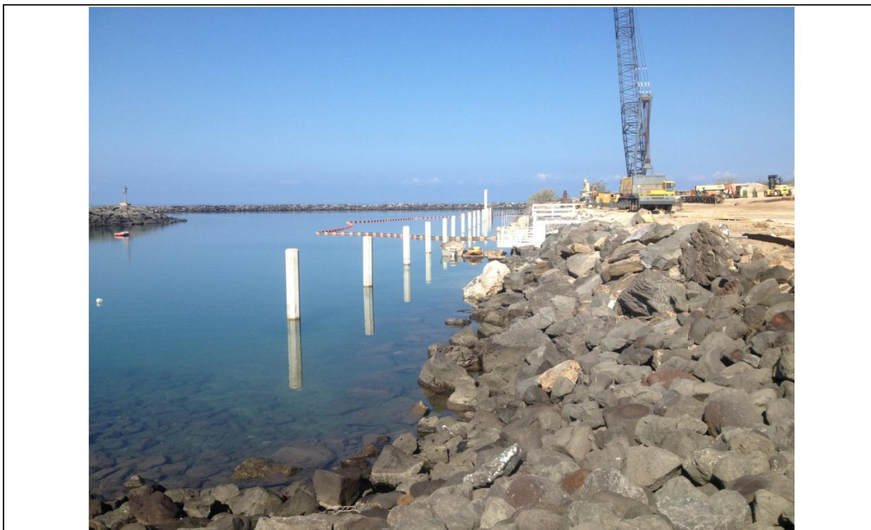
**Figure I.5-17 Pile Installation at Kawaihae Small Boat Harbor**
